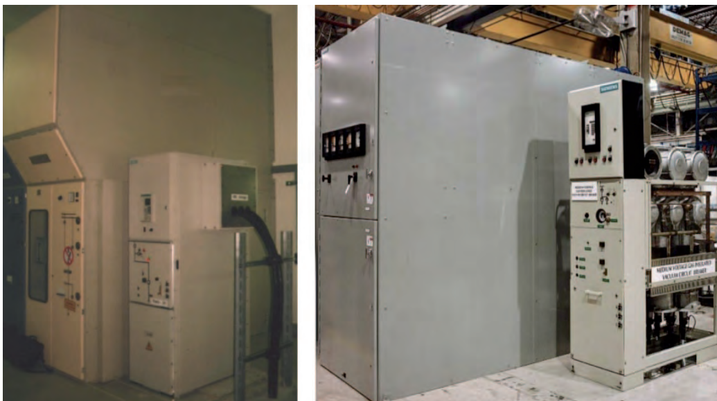
Figure 4 - Comparison between medium voltage air insulated switchgear (larger equipment on the left of each picture) and SF 6 switchgear (smaller equipment on the right of each picture). 24 kV switchgear (left picture), 36 kV switchgear (right picture).
