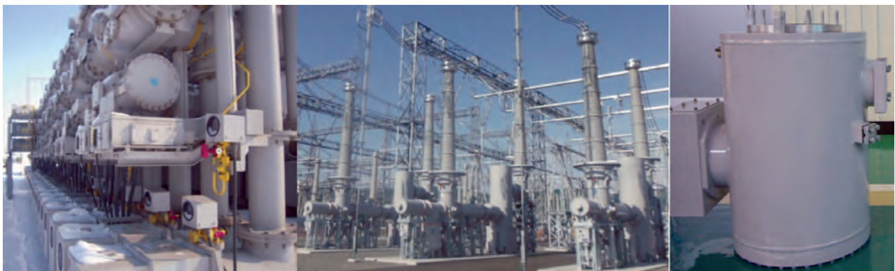
Figure 2 - 220kV GIS for TRANSELECTRICA, BRAZI VEST substation, Romania.
